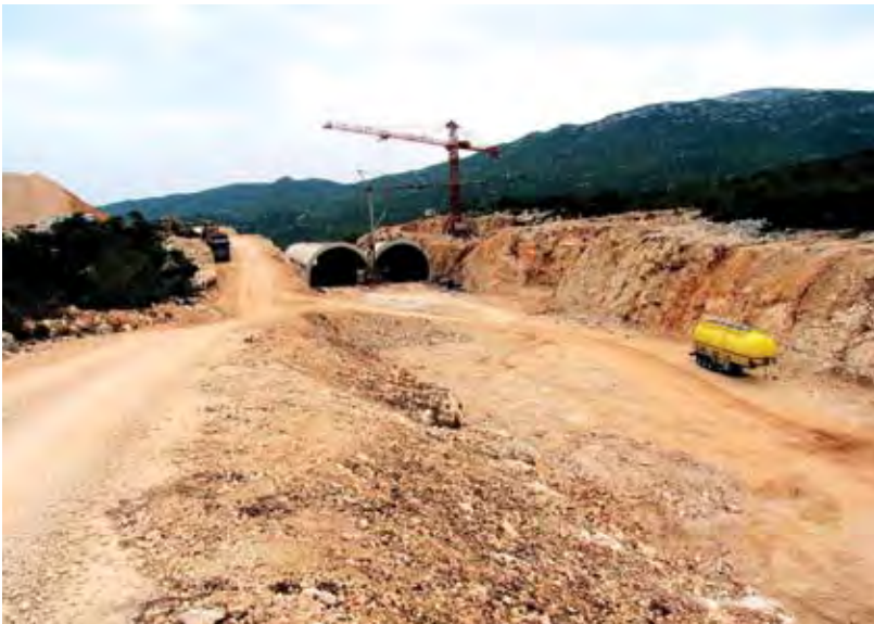
Fig 23 The Vrankovića ograda green bridge under construction (PHOTO BY J. KUSAK)
